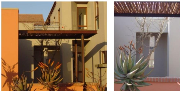
Pergola: Wattle laths contained in a frame
